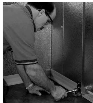
Attach slam brace with fastener provided
