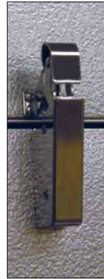
Spring actuated door closer
