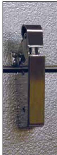
Spring actuated door closer
