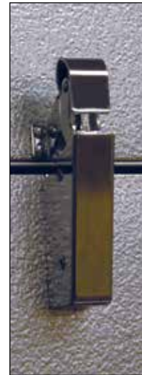
Spring actuated door closer
