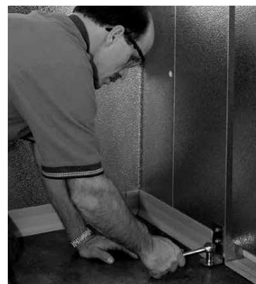
Attach slam brace with fastener provided
